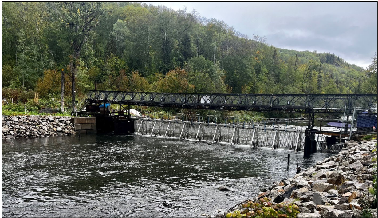
Upstream view of KSEF on September 17, 2024
