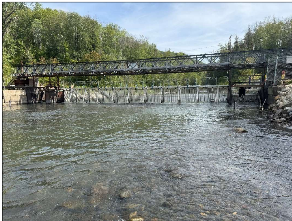
Upstream view of KSEF on September 3, 2024
