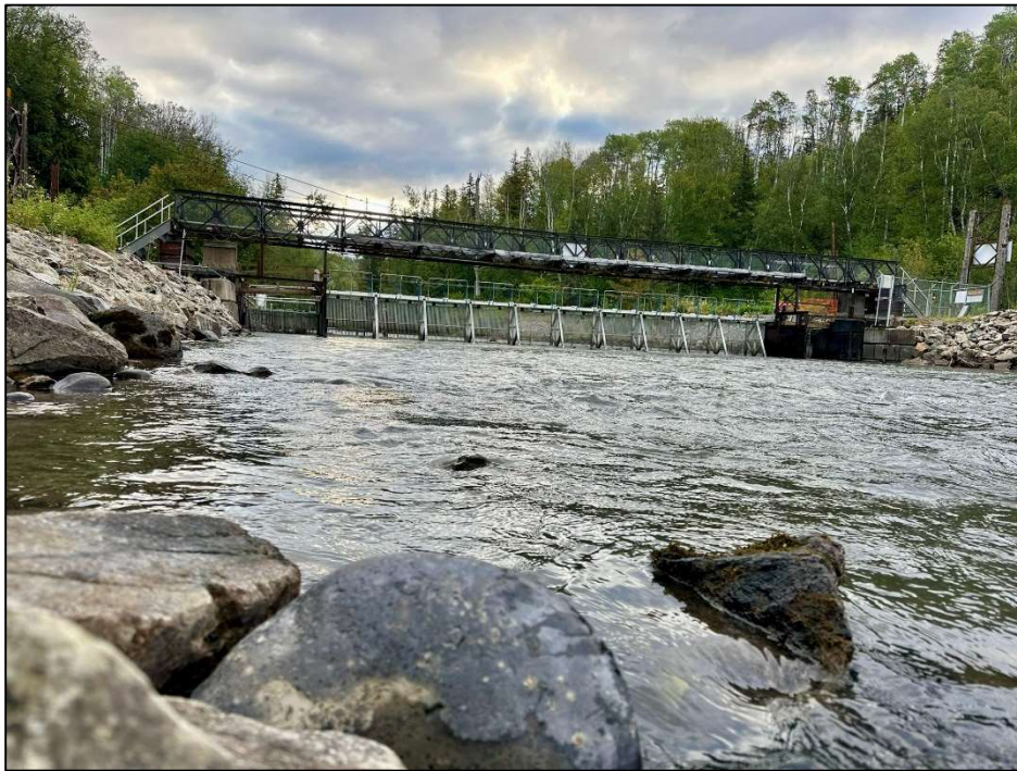
Upstream view of KSEF on August 27, 2024
