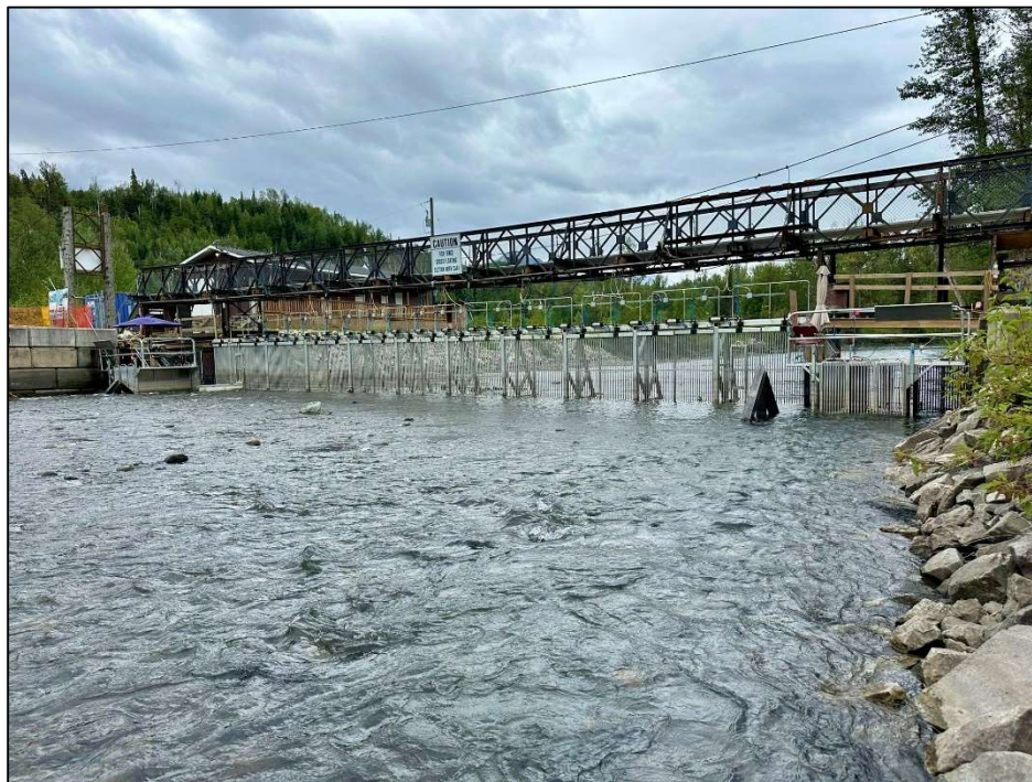
Downstream view of KSEF on August 20, 2024
